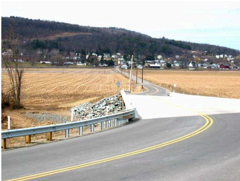
New Bridge Over Towanda Creek, Liberty Corners Road
